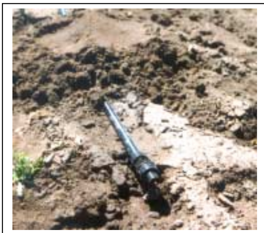
Close-up picture of automatic flushing caps. This cap requires 2.5 psi to close or almost 6 ft of head.
